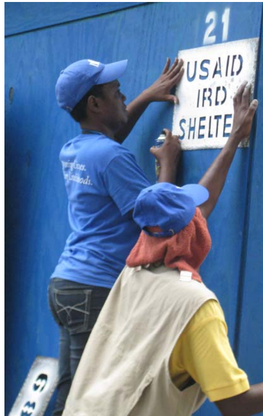
IRD plans to build 2,500 shelters by November. More than 140 are already completed.
