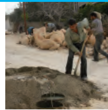
Mixing mortar for the main road
